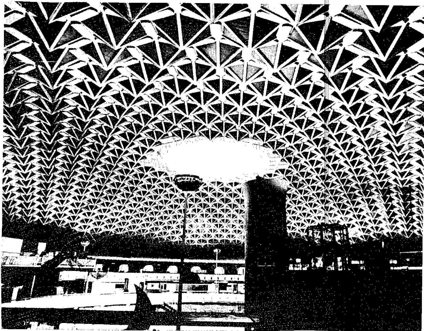
35. concrete air exhaust shaft
